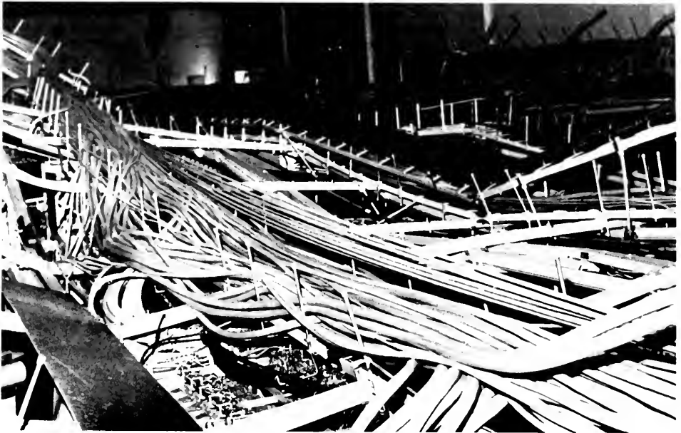
Photo 30. Sylmar Central Office. Collapsed automatic telephone switching equipment. General Telephone Company photo.
